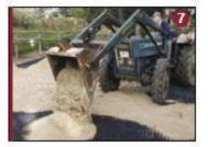
Fill in completely with pea gravel to ensure drainage in the stalls or use stone dust for turnouts.
